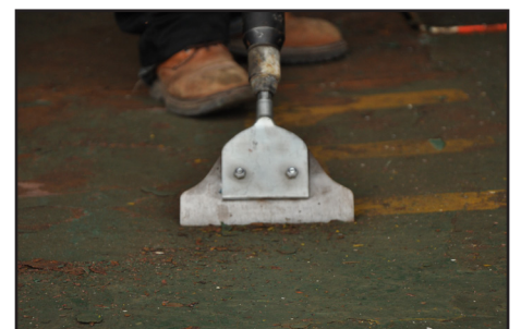
SHIP DECK RUST REMOVAL
